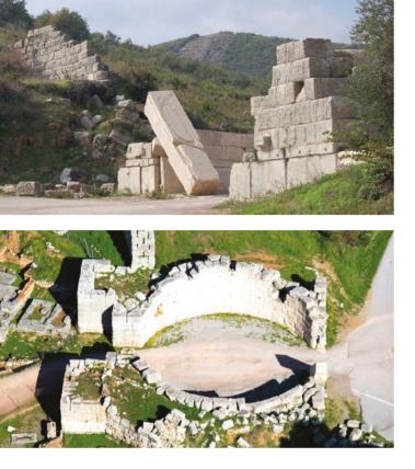
The strong exterior retaining wall of the Theatre is constructed with stone blocks imitating the fortifications. The retaining wall is interrupted at regular intervals by gates and staircases leading to the upper corridor. In the Roman period the Theatre was extensively repaired and acquired a threestoried stage.
